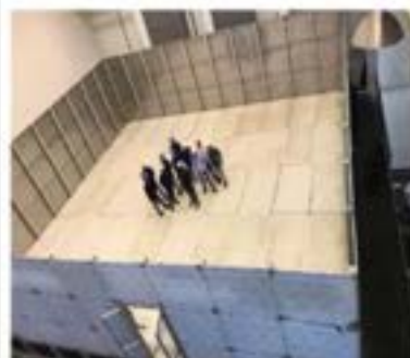
HIGH VOLTAGE DECK FOR INTERNATIONAL THERMO NUCLEAR EXPERIMENTAL REACTOR (ITER- INDIA)
